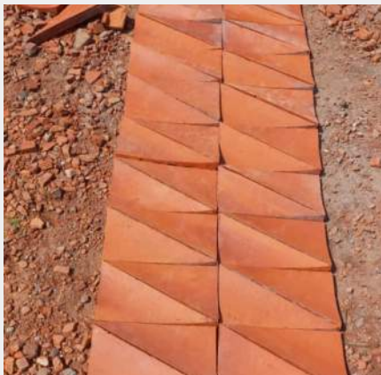
Test Bricks for the Exterior Facade at KSC
